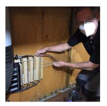
Thomas Rohlfs made good progress Wednesday, 11/18 and Friday, 11/20 installing the new capture system and completing the myriad wiring connections between the new stop tab units at the console, the capture system and the organ's new stop motors which had previously been installed in the organ case.
