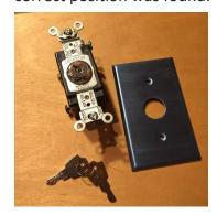
The old switch is being replaced by a new keyed switch from Leviton. The key and key slot on the new switch are readily recognizable. Inserting and turning the key results in a reassuring and audible click with the faithful Holtkamp organ powering on as it has for years at McAllister.
