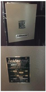
Tucked away inside the organ case. The old power supply is fed 240 volt-3 phase power and supplies the stop motors with 12-15 volt DC power.
