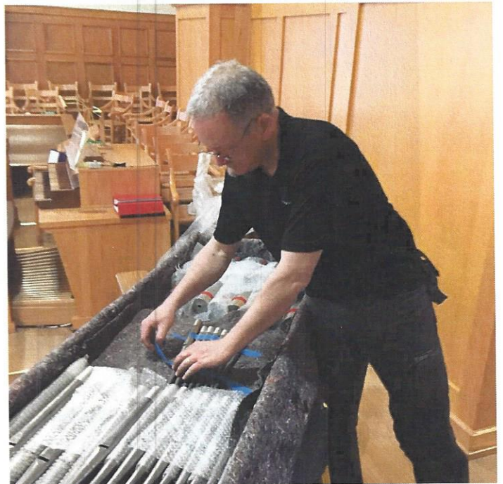
One of the wooden transport trays receives some of the last pipes removed from the Swell division of McAllister's Holtkamp pipe organ.
